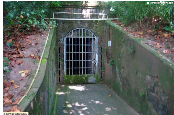
Site E: Tunnel
